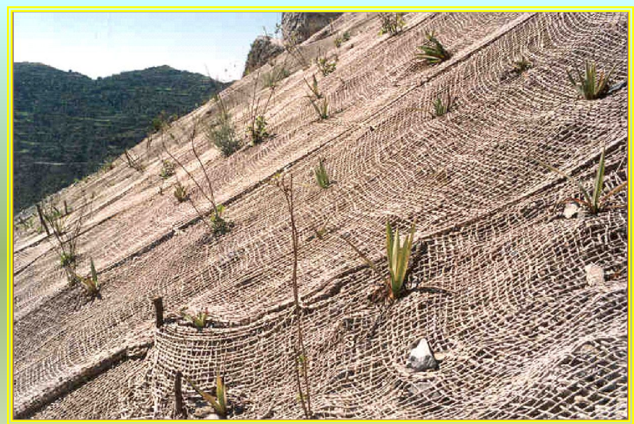
Geojute matting for slope stabilization
