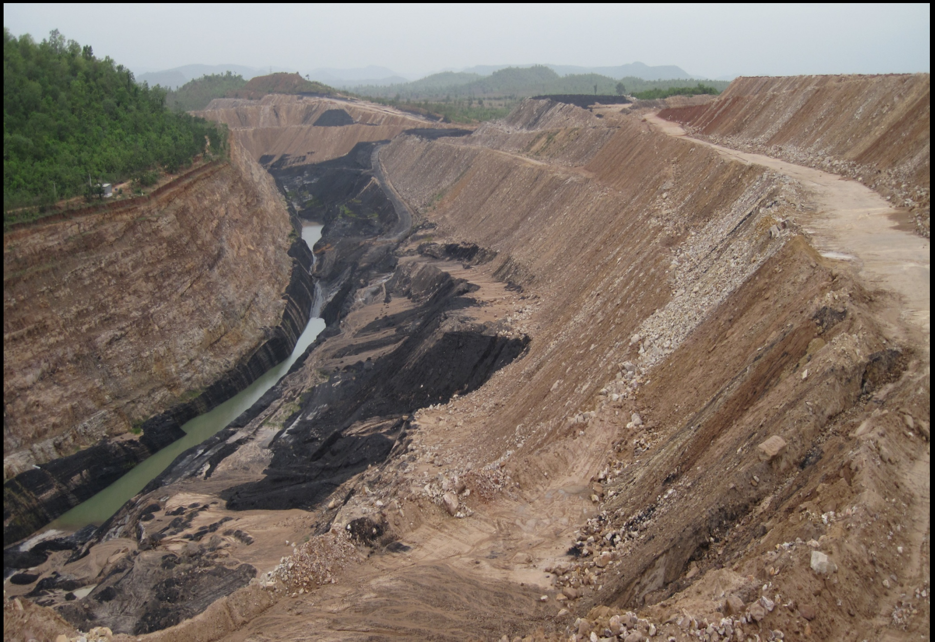
Back-filling of mined out soil into mine Pit-for rehabilitation
