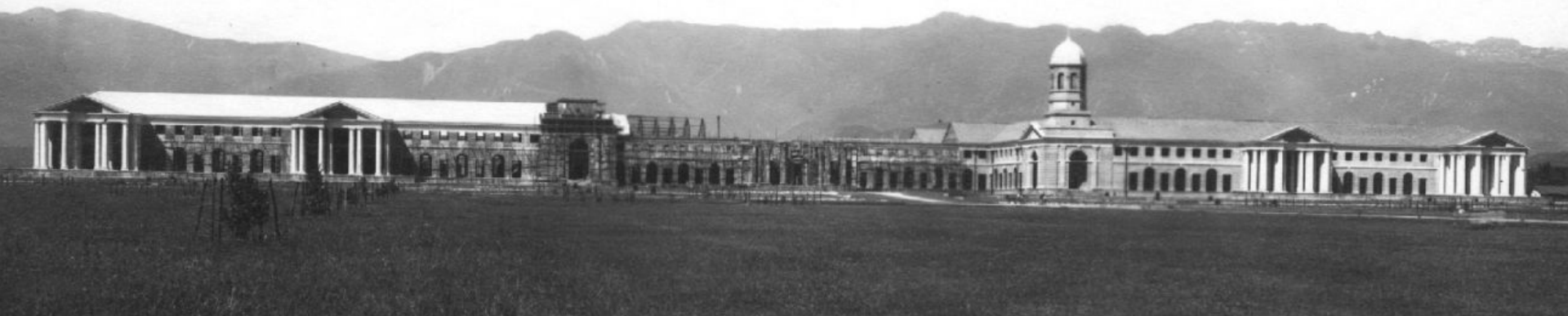
FRI building under construction: Photo: Har Swarup, 25.09.1927
