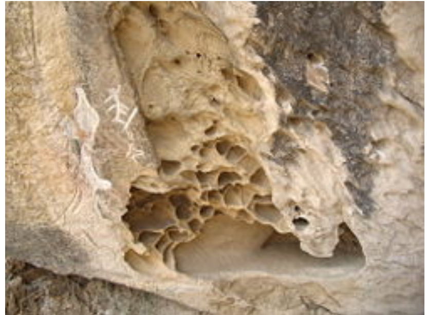
Weathering of Limestones
