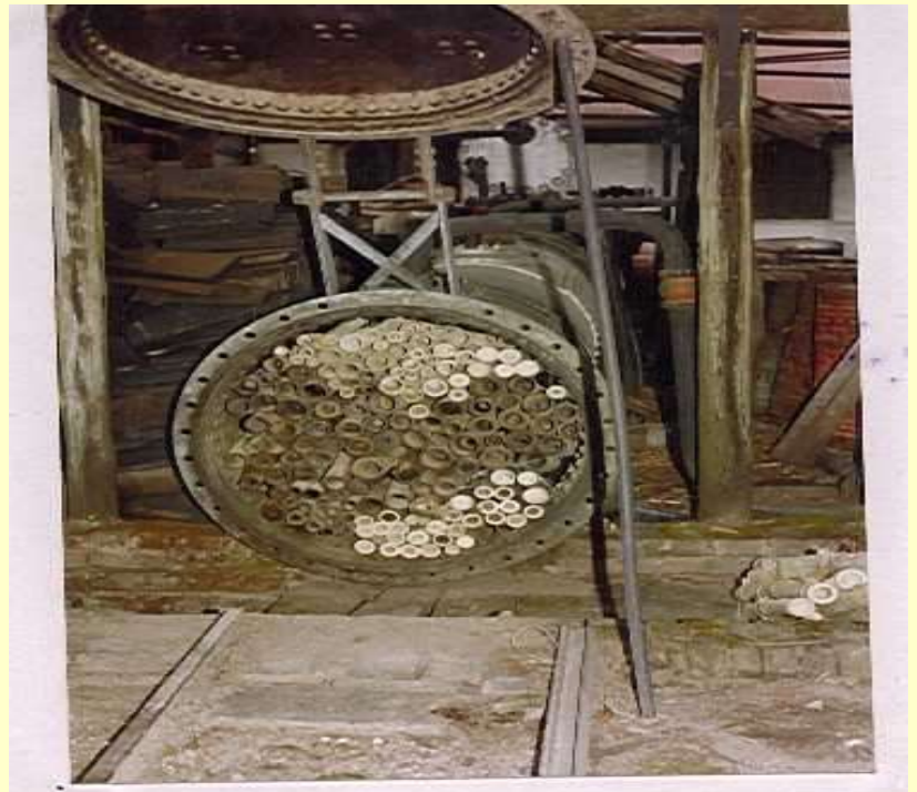
view of vacuum treatment plant for treating round or s...
