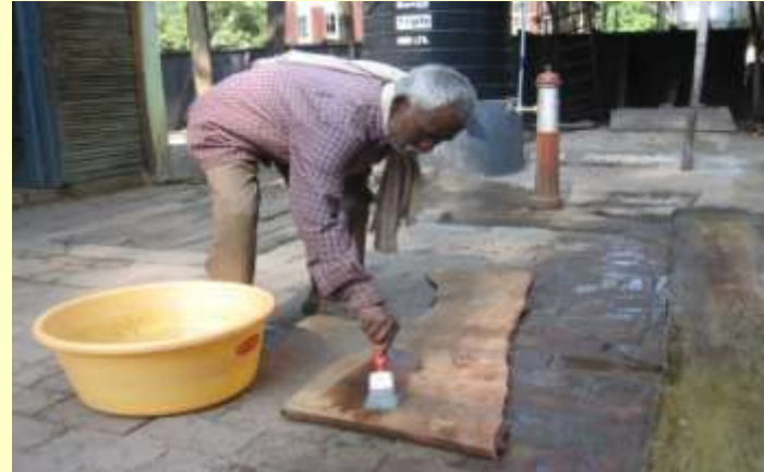
Preservative application through spraying/brushing
