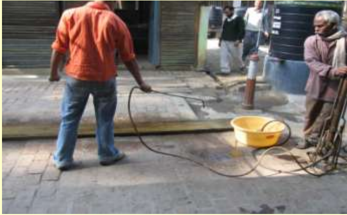
Preservative application through spraying/brushing
