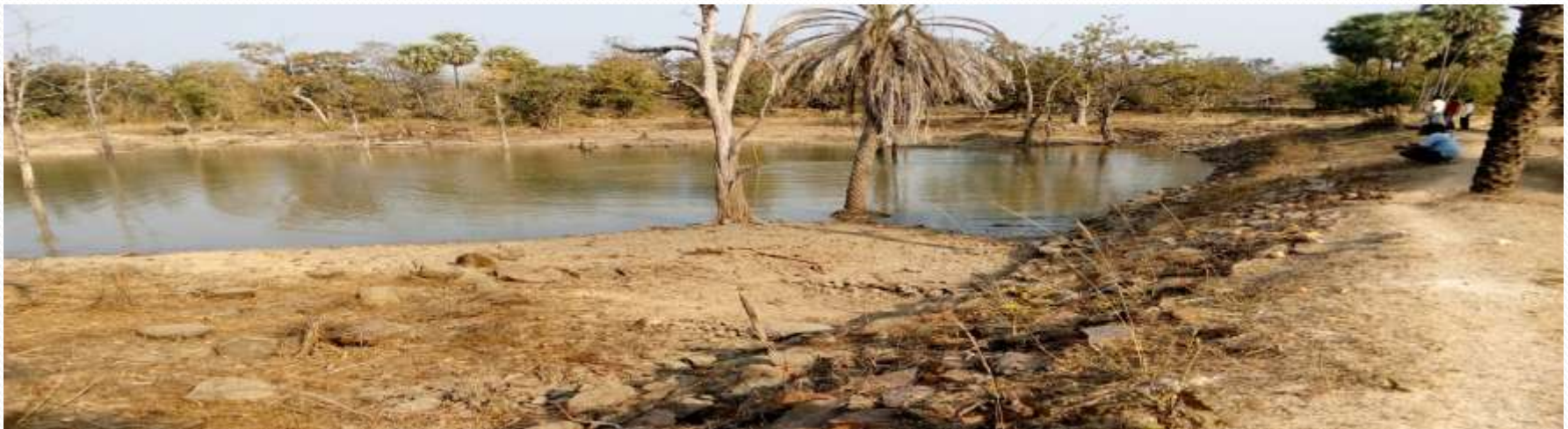
Figure 30- Construction of Nistari Tank and Nirmla Ghat at Gadiras Sukma.
