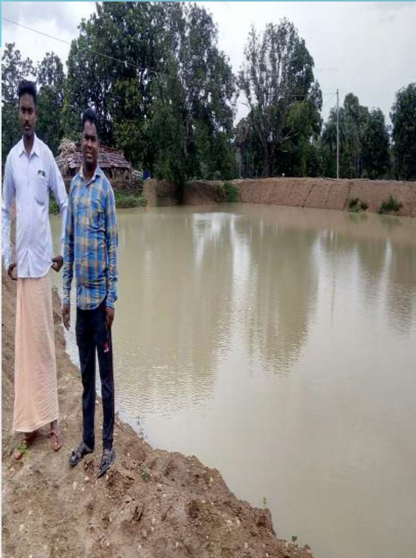
Figure 25- Construction of farm pond at Bodko, Sukma.
