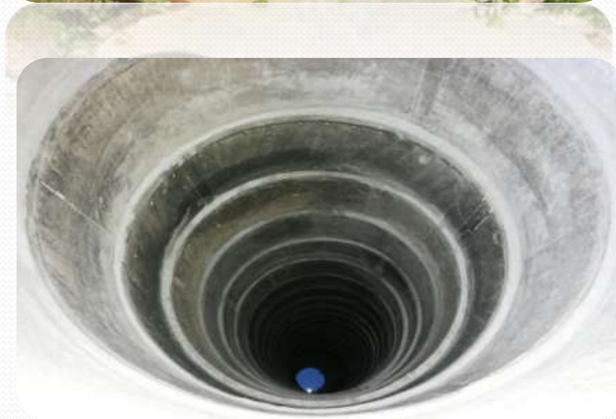
Figure 21- Construction of Dugwell at Birsathpal ,Chhindgarh.
