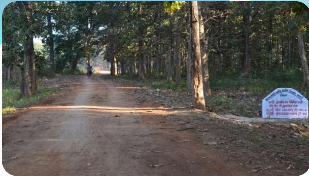
Gp- Pakela, Work- Muroom road, sanction amount- 9.88, Year- 2015-16
