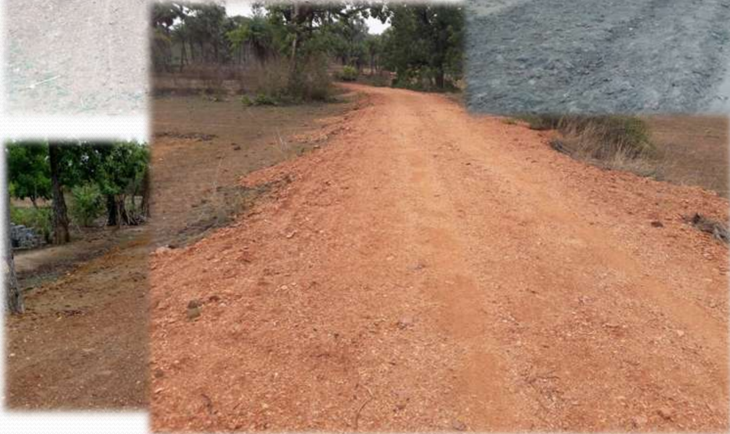
Figure 37- Construction of Earthen road at Budadi ,Sukma
