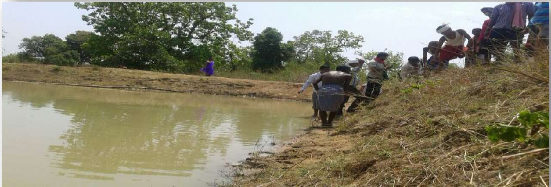
Figure 31- Construction of Nirmla ghat and Pond Clearance at Ramaram,Chickpal Sukma.
