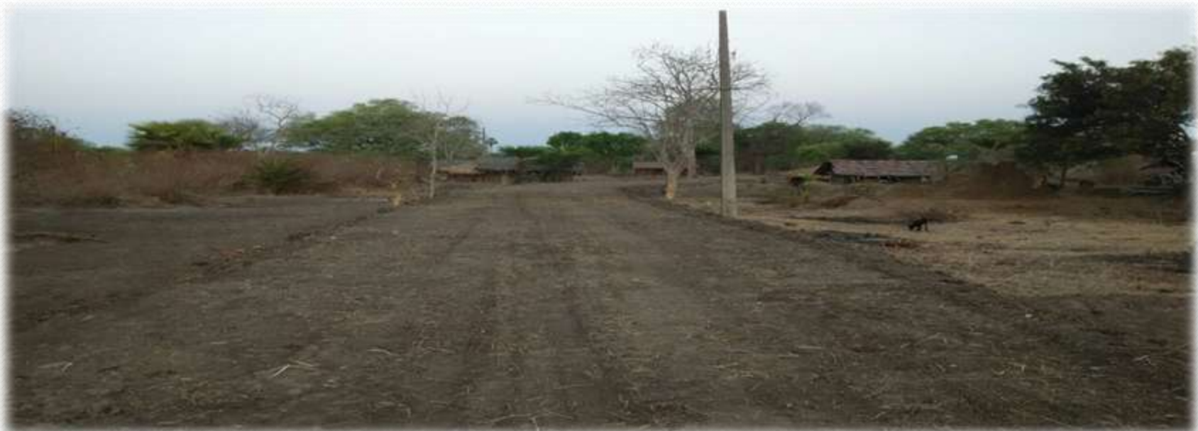
Figure 39 Construction of Earthen Road at BHEJJI, KONTA (AFTER)
