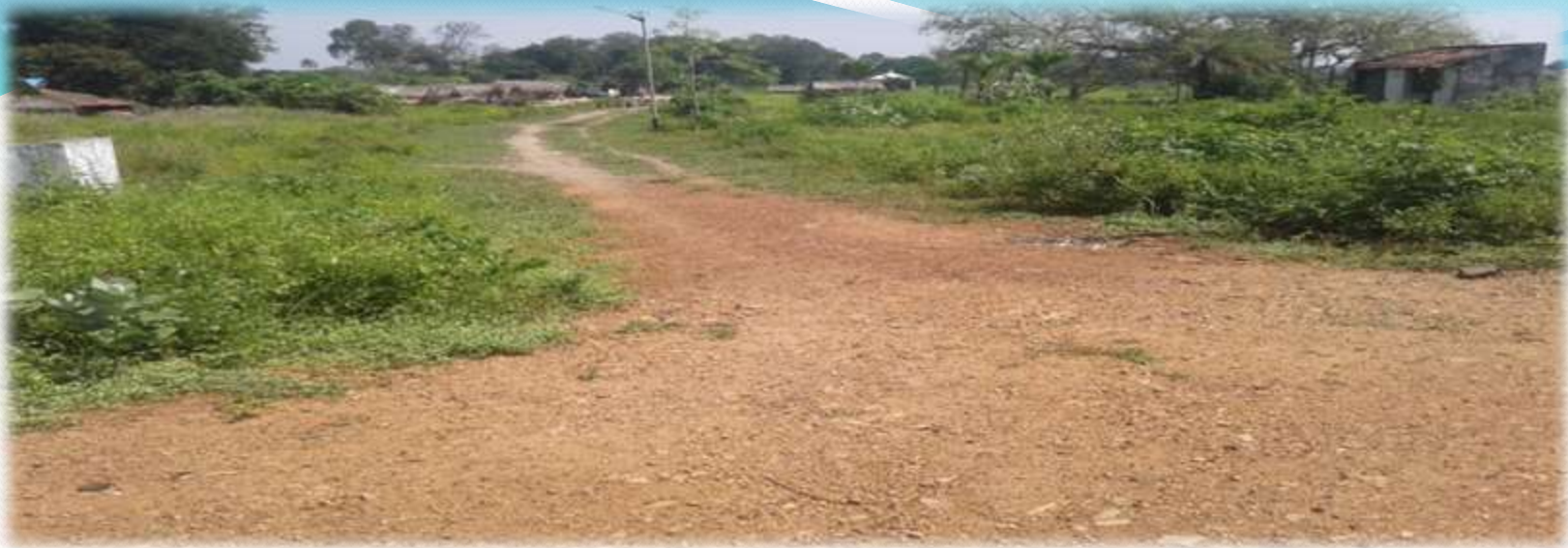
Construction of Earthen Road at BHEJJI, KONTA (BEFORE)
