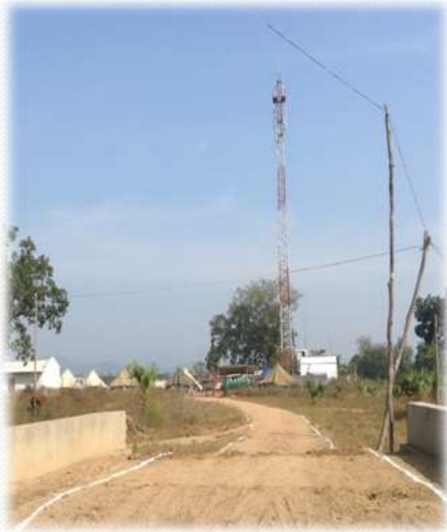
Installed Mobile tower in a village
