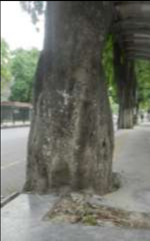
Restricted root space Cracks and insect attack
