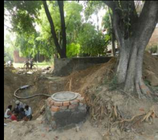
Active digging in CRR
